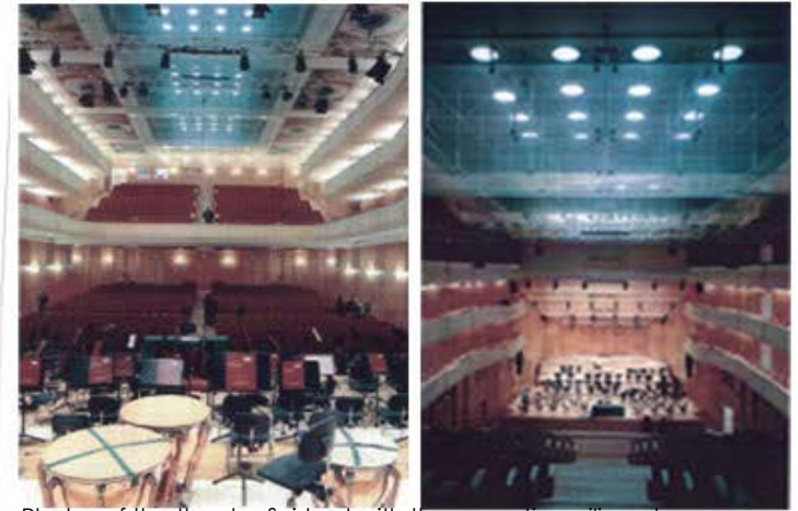
Photos of the theatre finished with the acoustic ceiling glass
